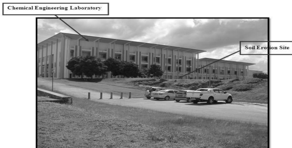
Figure 2: Soil Erosion Site Adjacent to the Chemical Engineering Laboratory
