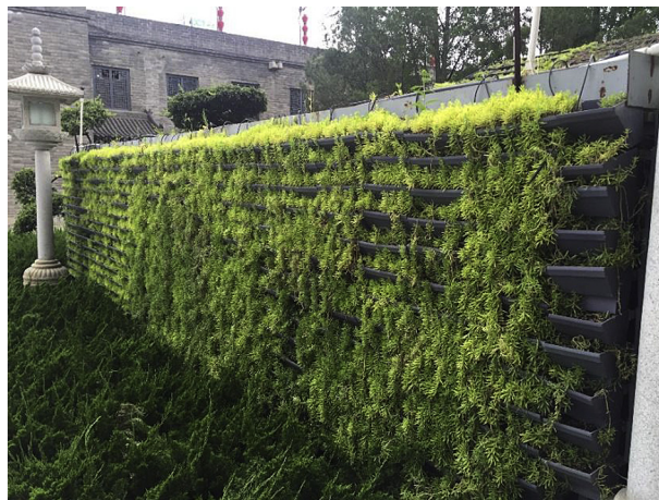
FIGURE 20.8 Modular box-type living wall in Xi'an, China.
