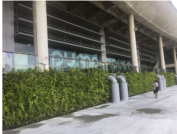
FIGURE 20.6 Living wall at the Marina Barrage in Singapore.
