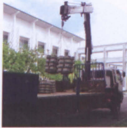
(a) Loading and unloading of StormPav blocks using lorry mounted crane
