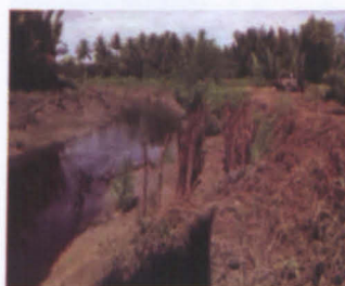
1) Installing bakau pile
