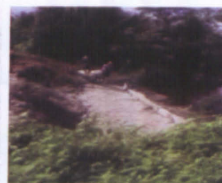
2) Stabilizing the lower berm
