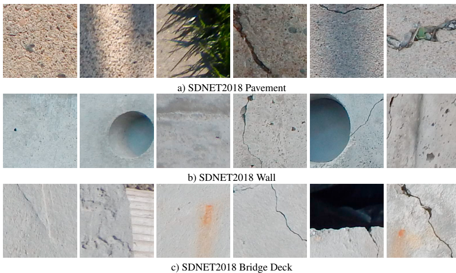
Fig. 2. Example of images from the “SDNET2018” dataset that contains three subsets with non-cracked and cracked pictures from three types of structures: a) pavement, b) wall, c) bridge deck.
