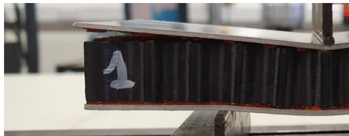
Figure 6.26 - Detail of failure between the core and upper skin during the beam flexure test
