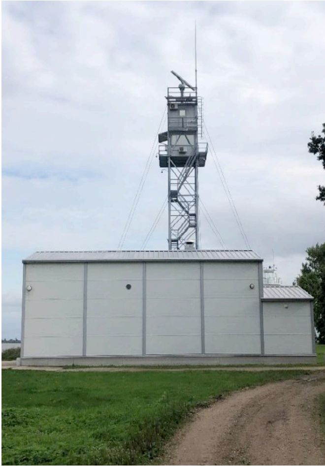
Figure 4: Photography of a the border guard building on the Peipsi Lake (source: Julien Gautier, 2021)
