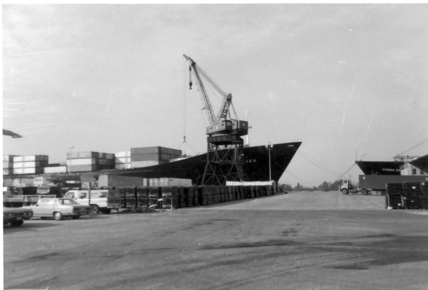
Figure 7: Gantry crane unloading the fore section of a container ship at Wilmington port.
