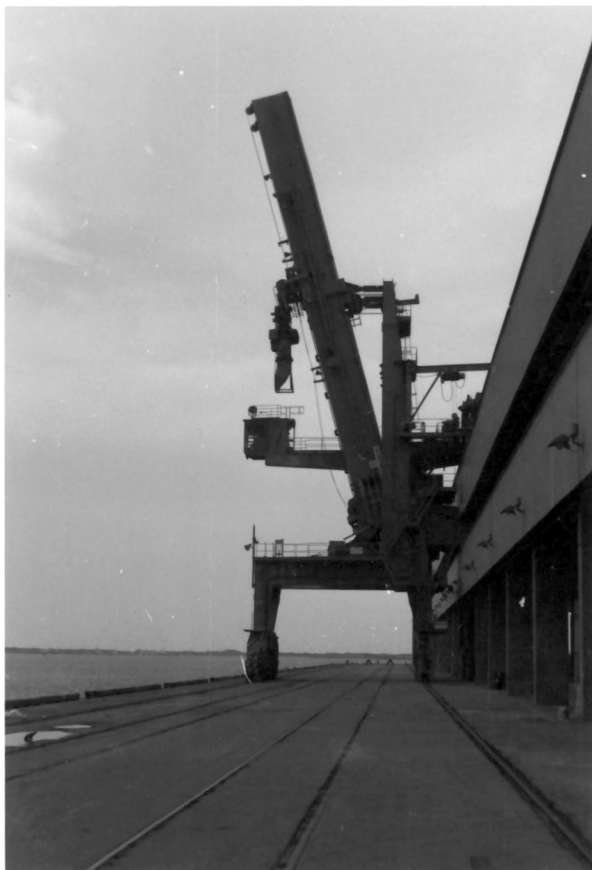
Figure 15: Dockside phosphate conveyor at the Morehead City port.
