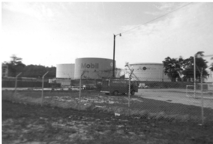
Figure 2: Private Petroleum storage facilities at the Wilmington port.
