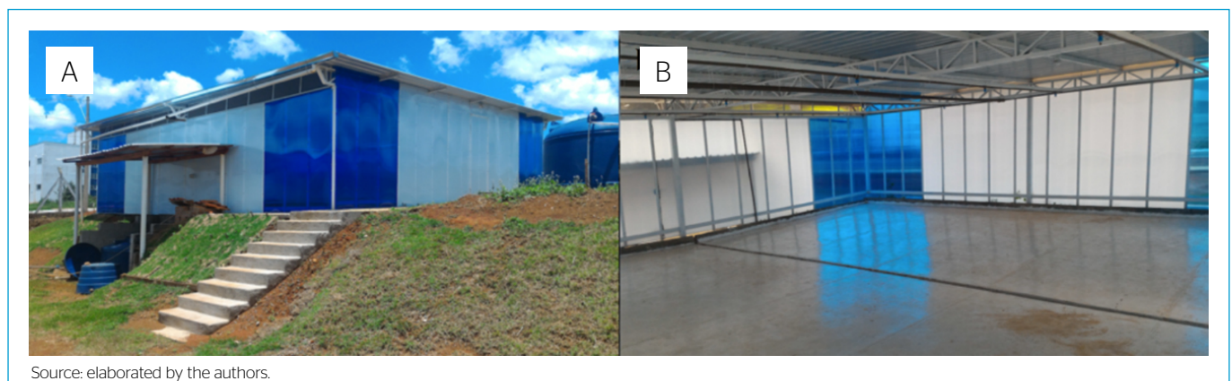
Figure 2 - Large-scale rainfall simulator (LSRS): (A) External view of the acrylic housing; (B) internal view, where it is possible to distinguish the concrete V-shaped surface and the light-steel structure to which the pipe network and nozzles are fixed.
