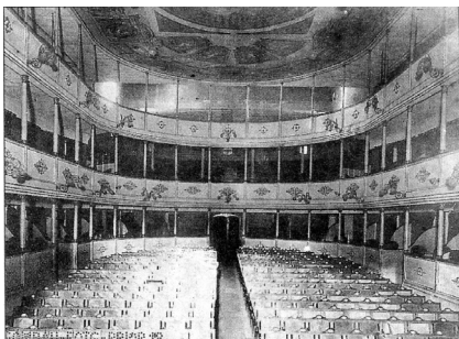
Fig.86 Interior teatro Liceo. V. Gombau
