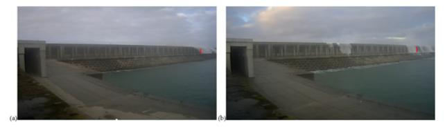
**Figure 8.** Aspect of overtopping event during (**a**) storm *c* and (**b**) storm *d* (monitoring section represented by a red line).
