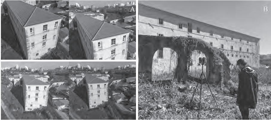
Fig. 1. (A) Imagery taken with Drone DJI – Phantom Vision 2; (B) Faro Focus 3D Laser Scanner.
