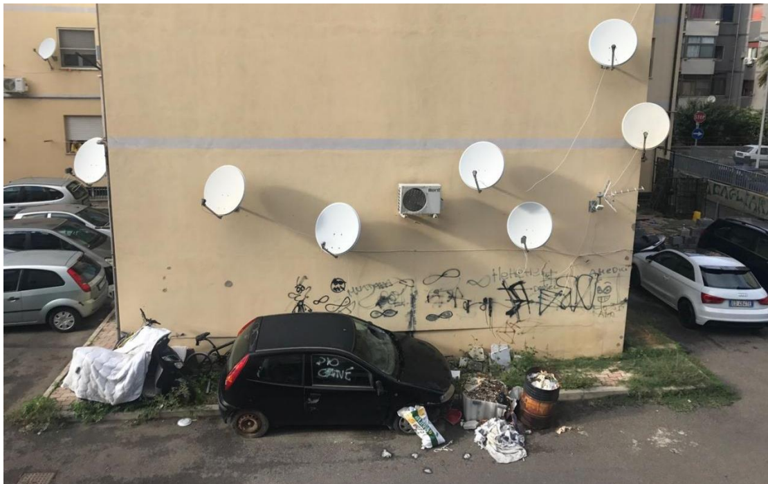
Figure 1.3 An unused area at the back of the building filled with waste (Author,2021)
