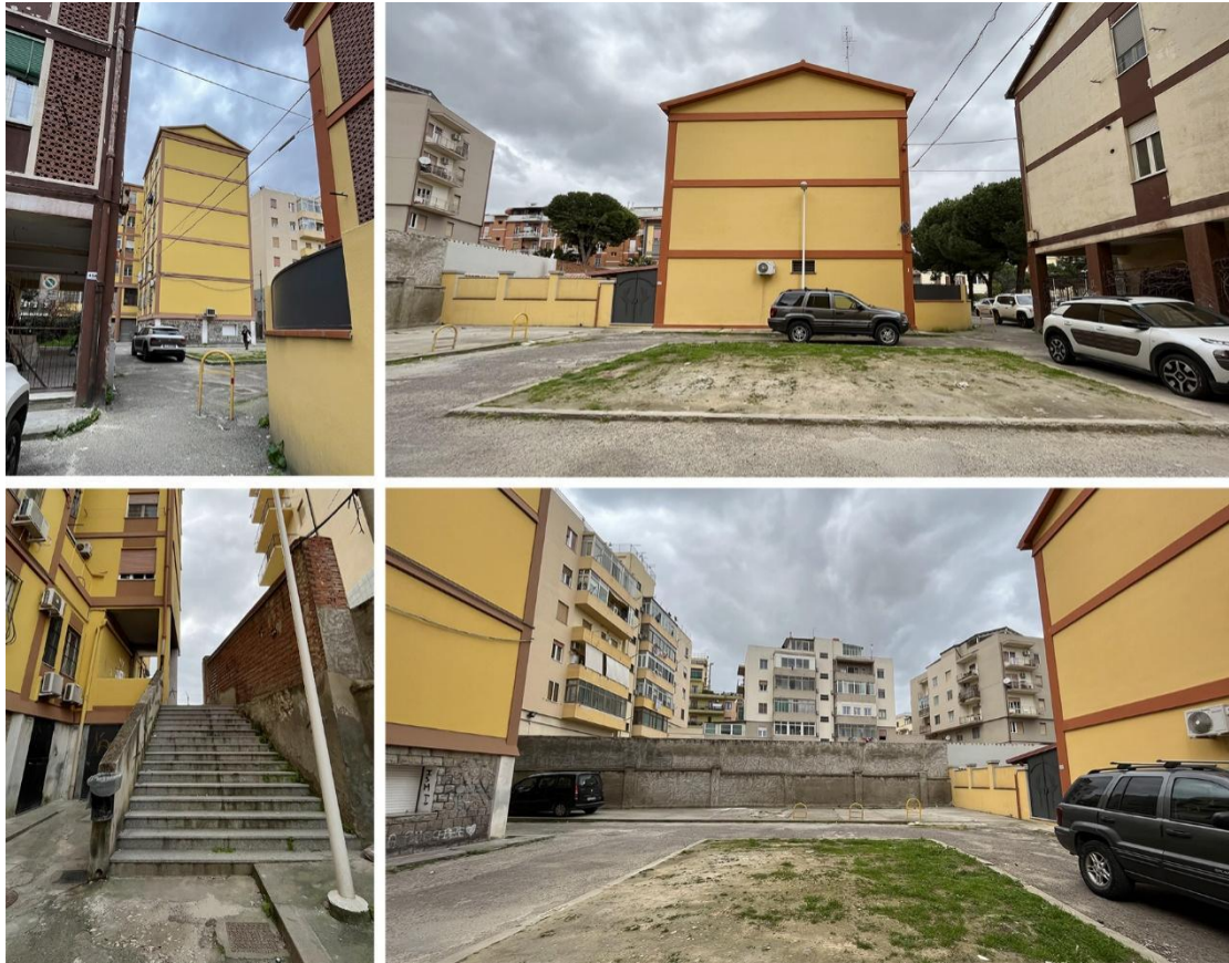
Figure 4.14 Photos of zone 8, Sparse landscaping and inefficient parking (Author,2022)
