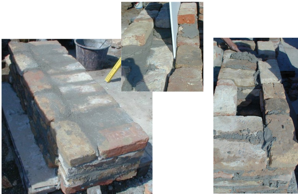
Photo 7. Construction of F4 test wall
