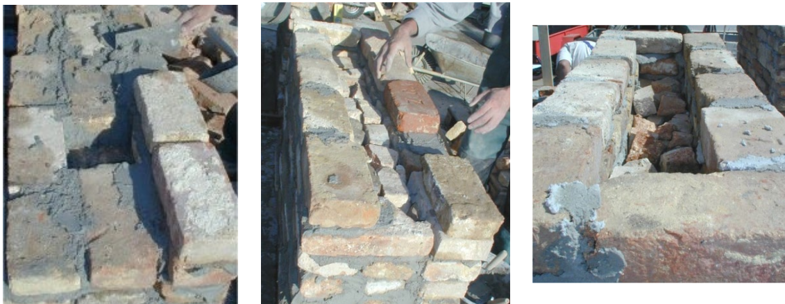
Photo 5. Construction of F2 test wall
