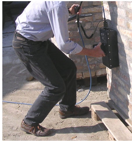
Photo 3. The GSSI 900 MHz antenna
