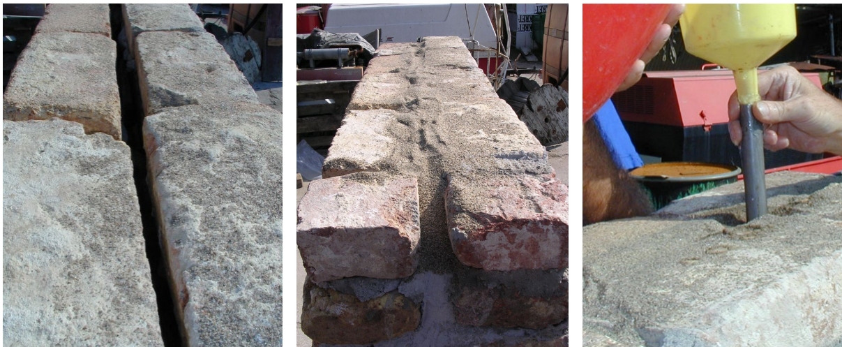
Photo 8. Left: air gap between the courses of F1 wall. Middle: the air gap is filled with sand. Right: the sand in the gap is wetted.
