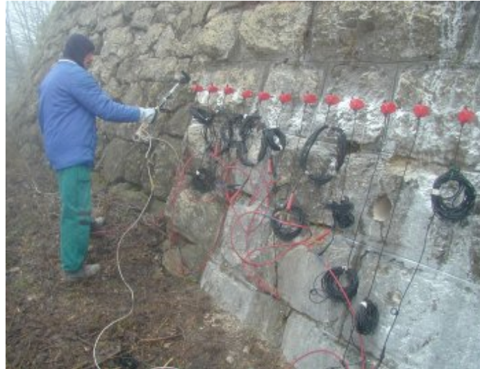
Image 8. Test configuration for the seismic investigation
