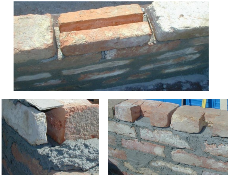
Photo 6. Construction of F3 test wall
