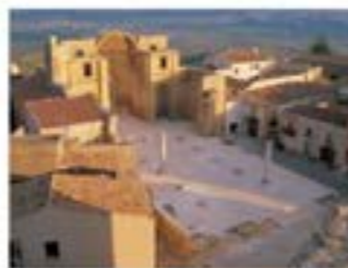
The conversion of the earthquake-devastated 17th-century church (Chiesa Madre) in Salemi, Italy, into a new urban plaza, dictates the addition of a new floor, circulation, structural improvements, and new lighting.
