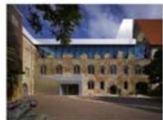
The Moritzburg Museum in Halle, Germany, is an example of a conversion from a semi-ruined roofless castle to a folding structural platform with the addition of a new roof and upper stories.
