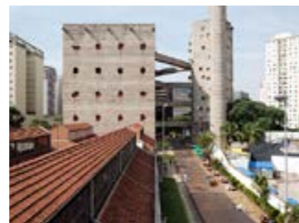
Lina Bo Bardi SESC Pompeia Factory 1977–1986 Industrial Factory a public place for entertainment and education archaeological excavations.
