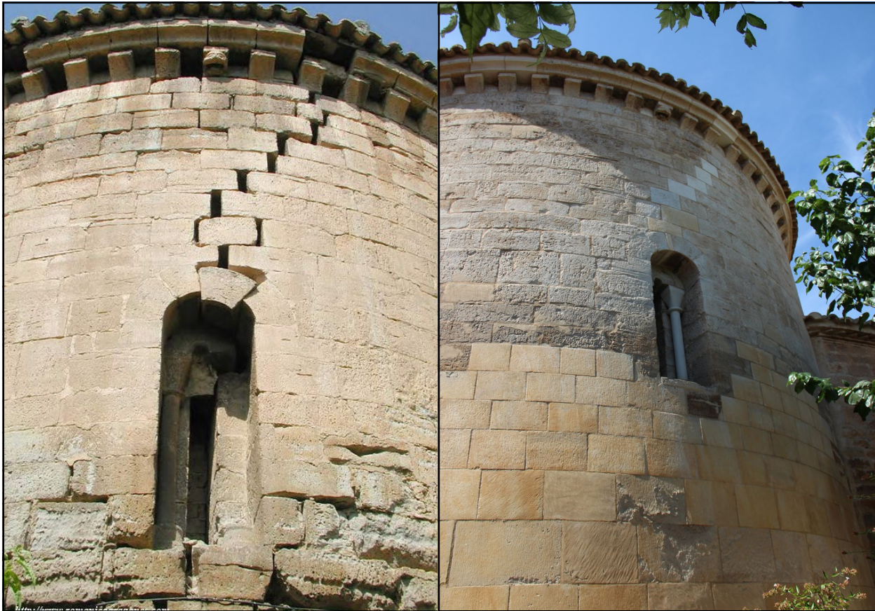
Figure 5. (a) Church of Nuestra Señora, Ballobar (Huesca), before its restoration (Source: Románico Aragonés http://www.romanicoaragones.com/33-Bajocinca/Ballobar%20g04.jpg ) (b) Church of Nuestra Señora, Ballobar (Huesca), after its restoration. (Photo by María Teresa Chicote Pompanin)
