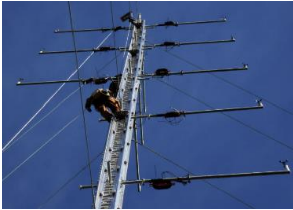
(a) Tower for data observation
