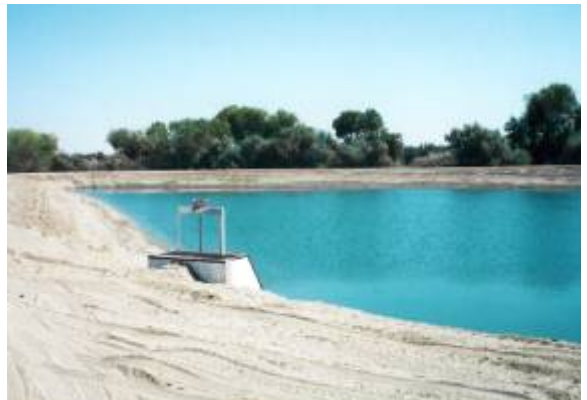
Figure 1. Gravity in – gravity out reservoir constructed to store water for use during the peak period
