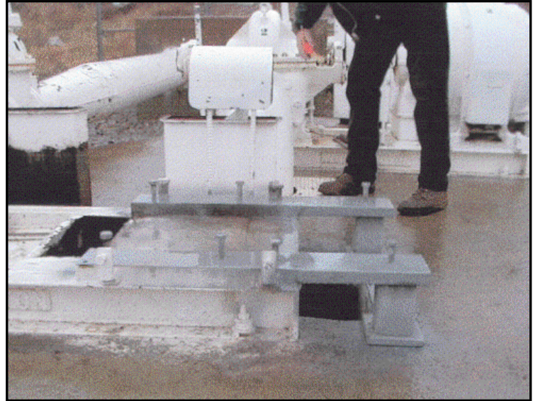
Figure 3. Motor Stand Modifications at Roza I.D. (Photo courtesy of Roza I.D.).
