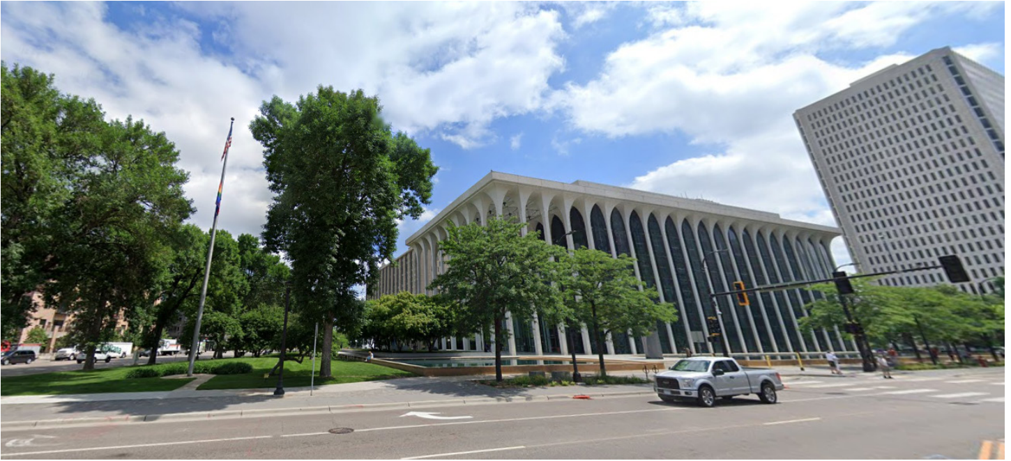
View to the north of the site.
