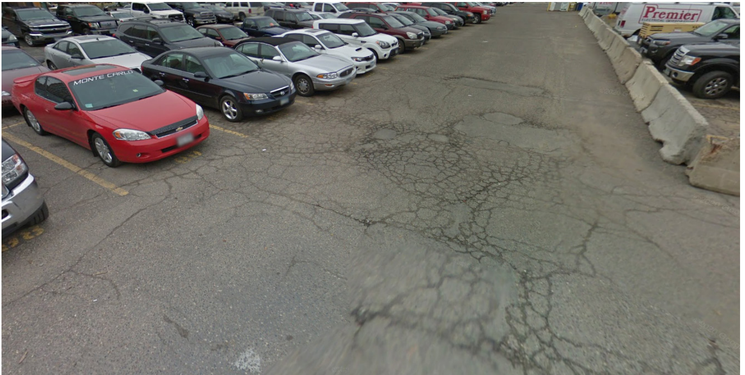
View of Parking Lot on Site
