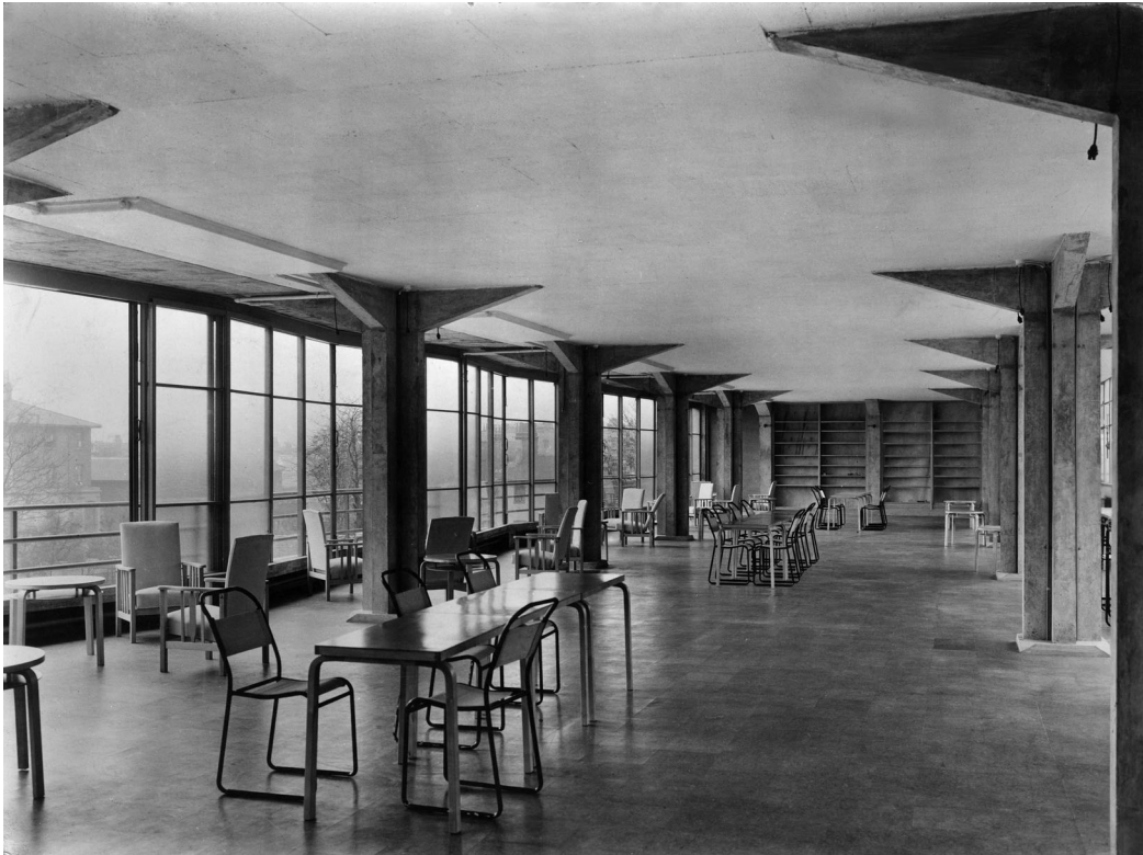
Figure 4. The Lounge and Library of the Pioneer Health Centre with views of mushroom columns, 1935 (Architectural Press Archive / RIBA Collections).
