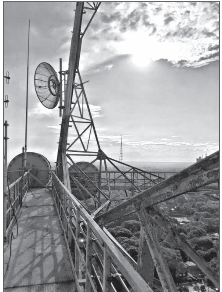
Figure 3 — The Willoughby tower looking back toward Artarmon Triangle tower. This picture illustrates a series of antennas mounted in just one section of the tower (Photograph taken by the study researcher).
