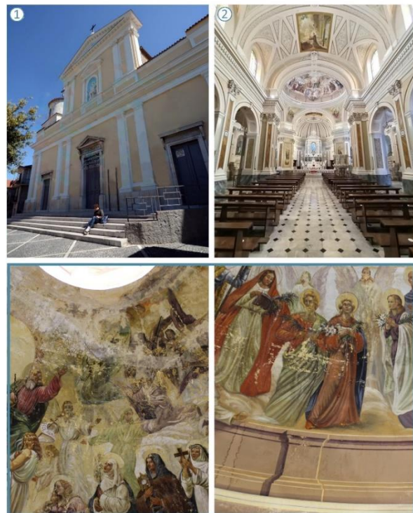
Figure 1. Church of San Michele Arcangelo in Padula. Plan and photographs of the façade and interior. Detailed images of the damaged frescoes of the dome.
