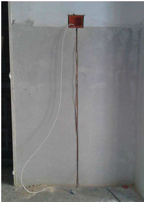
Fig. 4. Installation of the SE and installation of the wall box.
