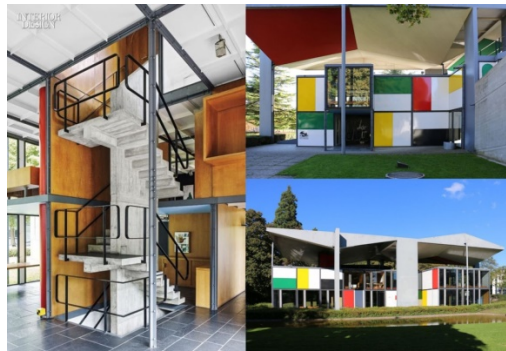
Fig. 7: Interior and exterior of the Maison de l'Homme
