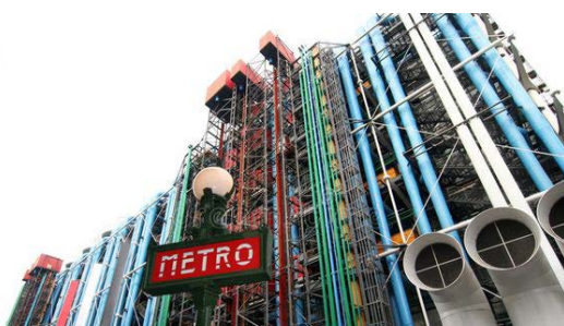
Fig. 11: facade on rue beaubourg
