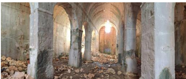
Figure 3. Interior view of Akkale Cistern
