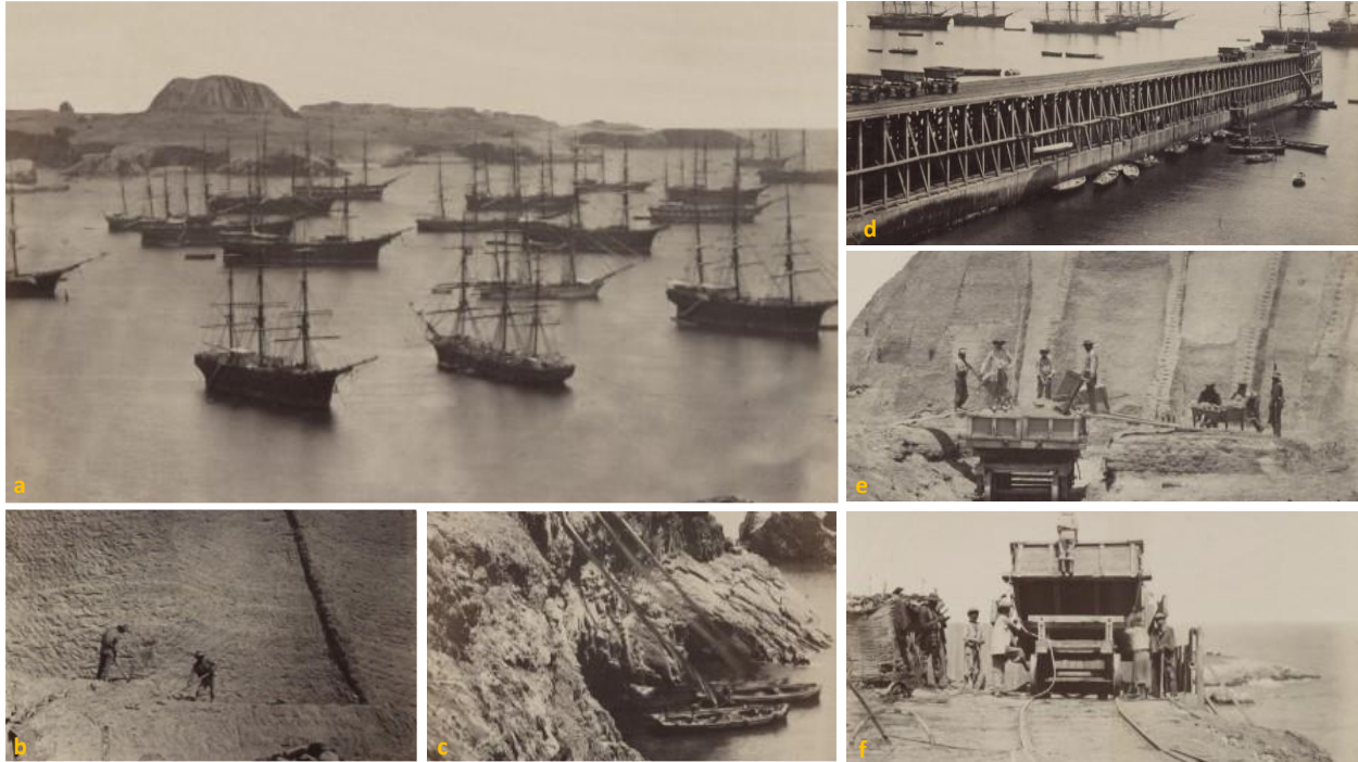
Figure 5.4. Guano extraction at the Chinchas, 1865. (a) “North Island, Chincha Islands, With Part of Fleet Waiting For Guano.” (b) “Strata of guano, Chincha Islands.” (c) “Shoots for loading the lighters with guano, Chincha Islands.” (d) “View of the Great Pier, With Shipping Waiting For Guano.” (e) “Loading cars with guano at the great heap, Chincha Islands.” (f) “Emptying Cars of Guano into the Shoot.” All pictures by H. Moulton (negative). Positive by A. Gardner. All pictures taken from: Gardener, Alexander, and Henry De Witt Moulton (photographer). 1865. Rays of Sunlight from South America . Washington, D.C.: Philip & Solomons.
