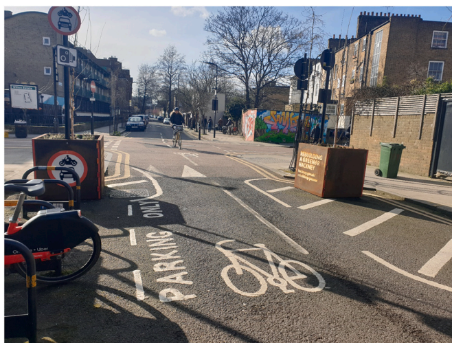
Fig. 1. Modal filter in Hackney, East London (sign with red border indicates 'no motor traffic'). Those in private cars can drive up to the filter on each side but not pass through it).
