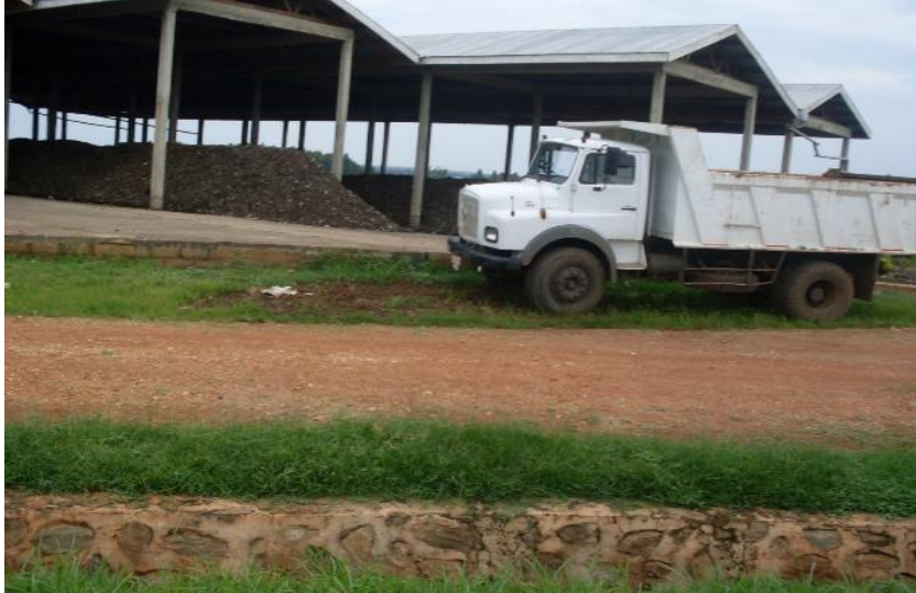
Figure 0-1 Mbale Municipal Composting plant. Source: Mbale Municipal
