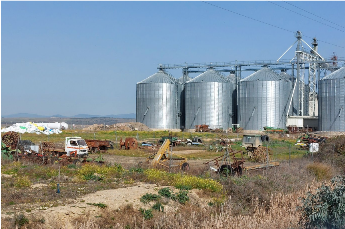
Rice silos and old rusty equipment for rice cultivation nearby Palazuelo
