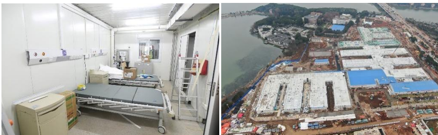
Figure 9. Huoshenshan Field Hospital ventilation system-left ( Mcdonald, 2020 ) and blue anti-seepage membrane-right ( Zhang, 2020 )
