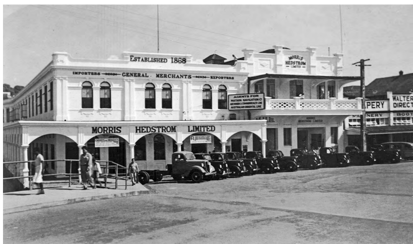
Figure 15.3: Morris Hedstrom building next to Nabukalou Creek, n.d.
