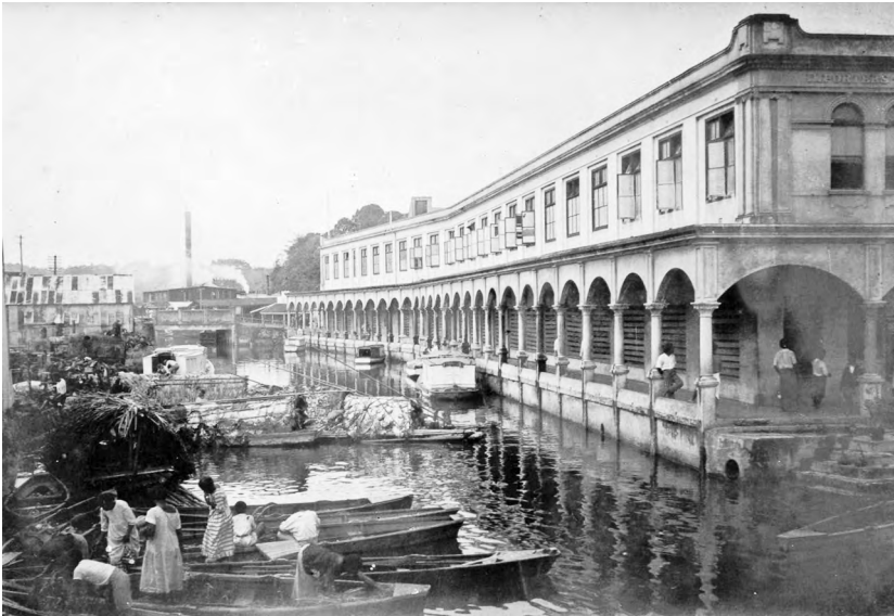
Figure 14.2: Nabukalou Creek, n.d.
