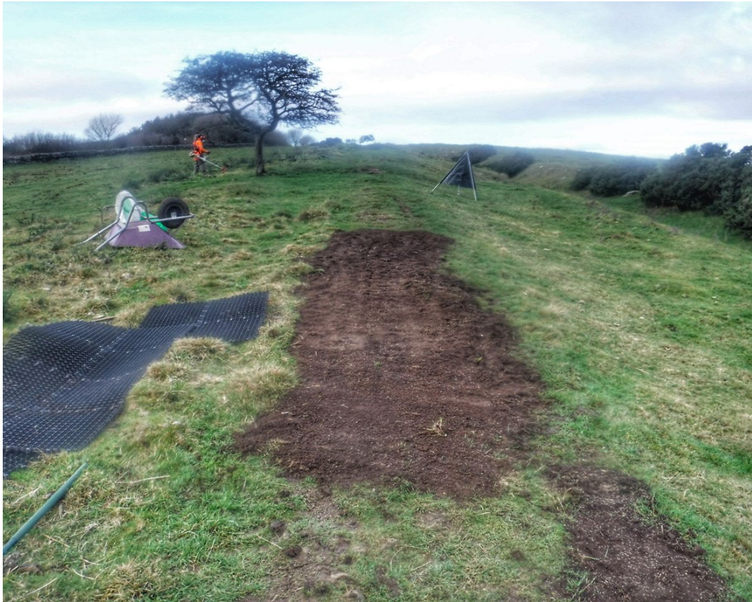
Figure 12: Soil is collected from molehills and mixed with grass-seed to repair the erosion. © Northumberland National Park
