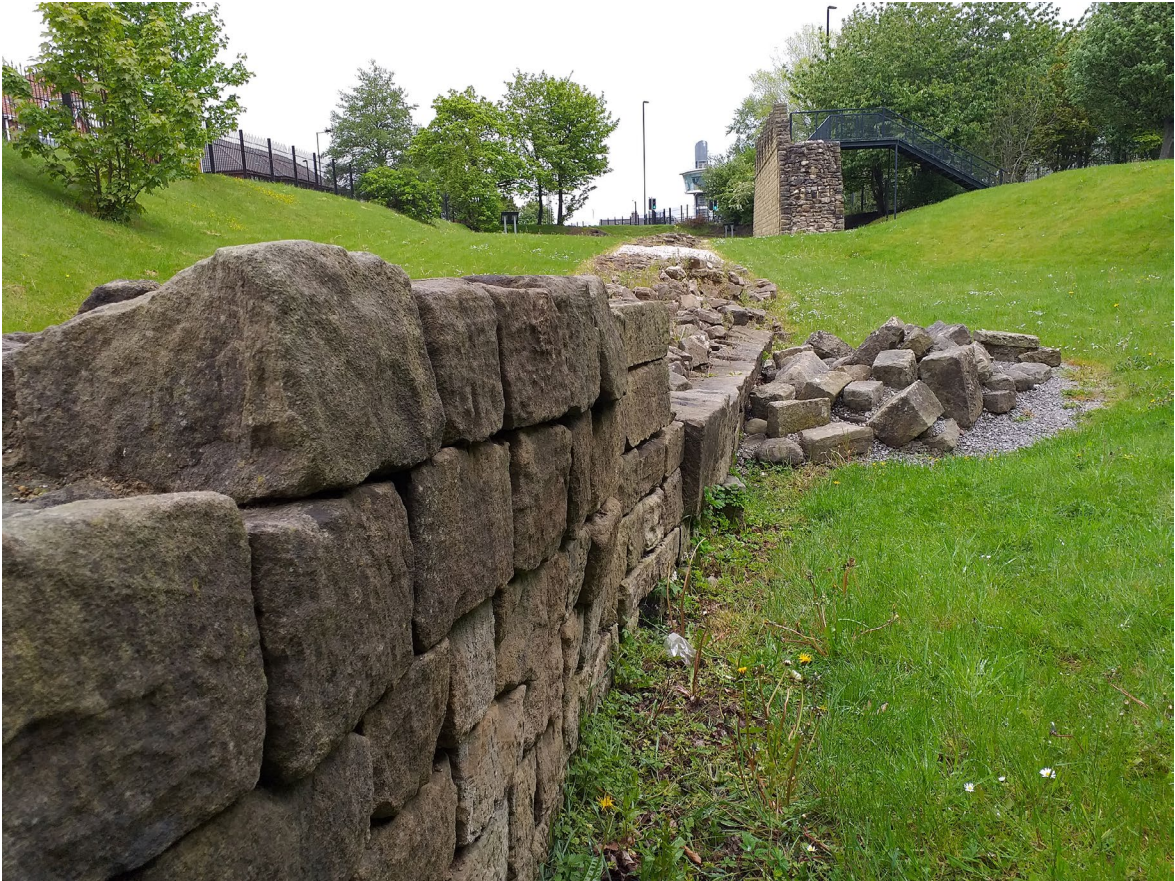
Figure 1: The excavated remains of Hadrian's Wall at Segedunum with the reconstructed section of Wall beyond. © Geoff Woodward
