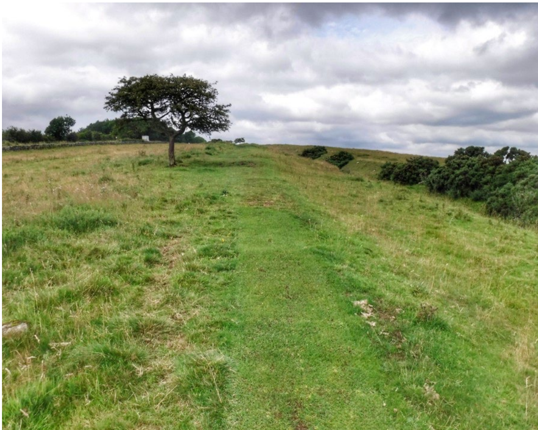
Figure 14: The membrane is removed once the grass/repair has become durable enough to withstand usage. © Northumberland National Park
