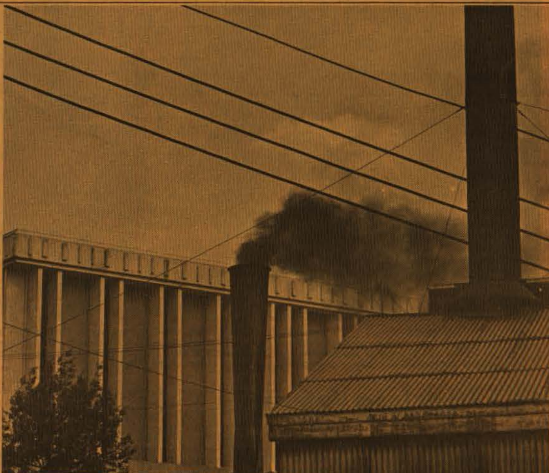
SMOKE POLLUTING AIR . . . . Although Murray isn't a large city by any means, it's beginning to look and smell like a large industrial area at times. The 45-year-old campus heating system, located behind the Science Bldg., spews out black coal smoke which is giving many people a right to
