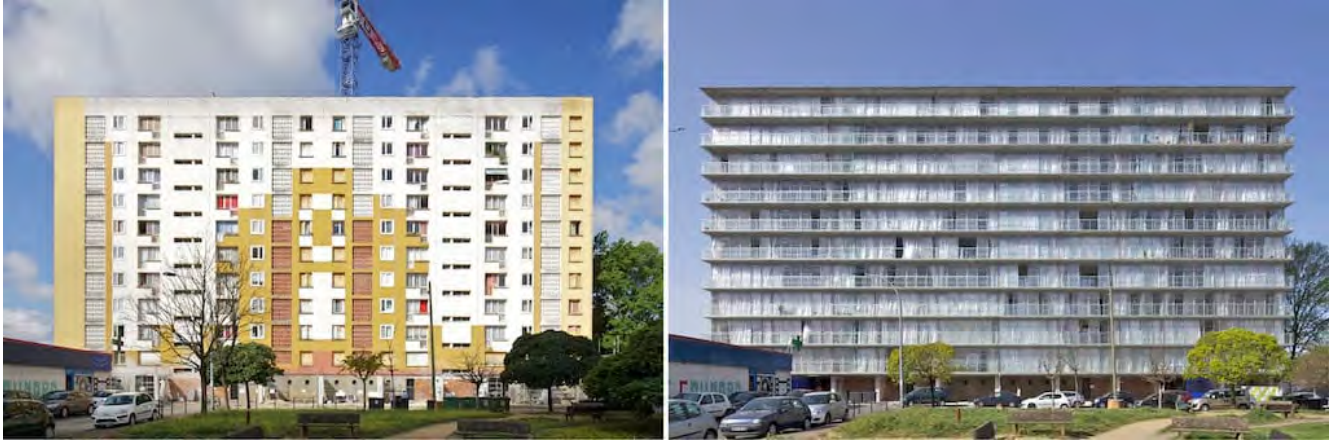
Figure 0.8, Lacaton & Vassal, Transformation of 530 Dwellings , 2016,
