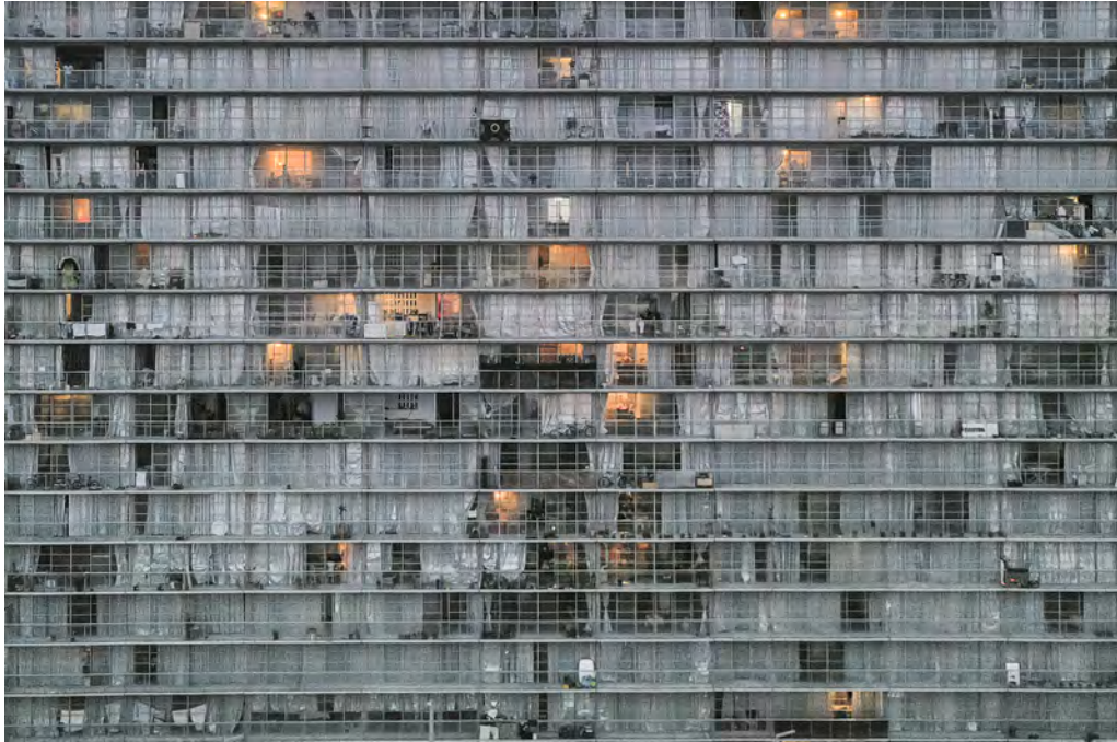
Figure 0.4 , Lacaton & Vassal, Transformation of 530 Dwellings , 2016,
