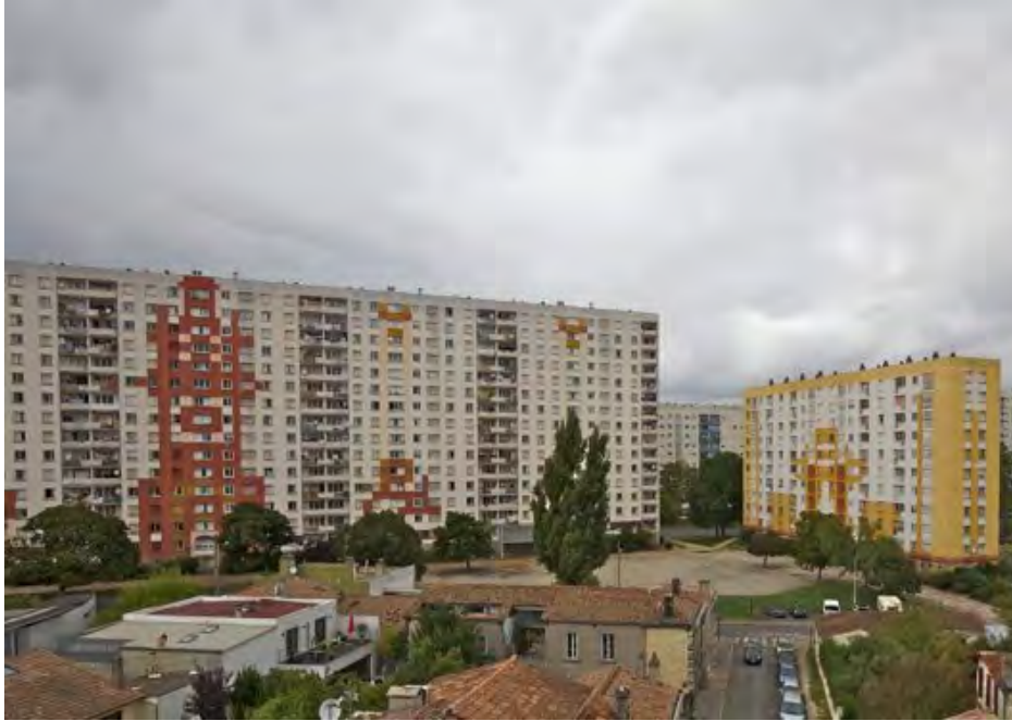
Figure 1.14 , Lacaton & Vassal, Transformation of 530 Dwellings , 2016,
