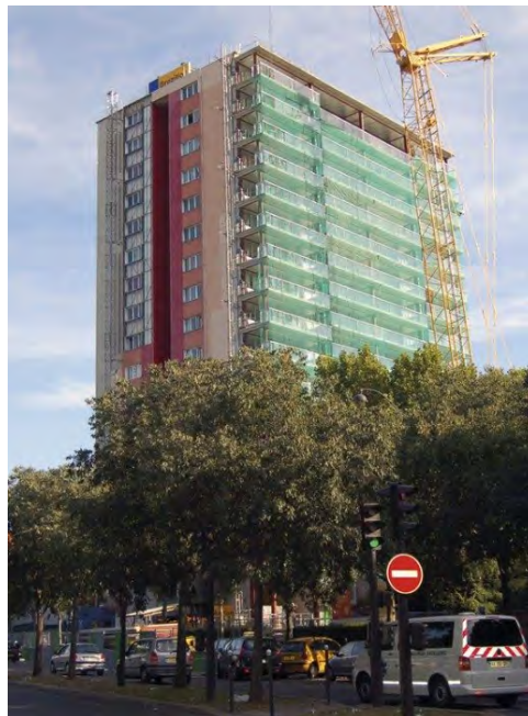
Figure 1.5 , Lacaton & Vassal, Transformation of the Bois le Prêtre Tower , 2011, https://www.archilovers.com/projects/74486/tour-bois-le-pretre.html
