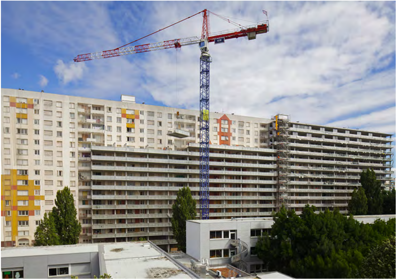
Figure 0.2, Lacaton & Vassal, Transformation of 530 Dwellings , 2016,
