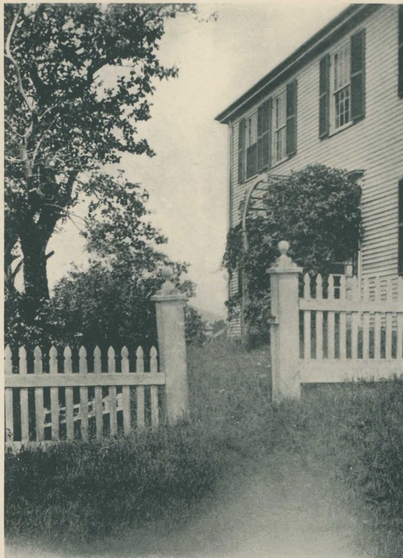
Detail of Main Façade.
