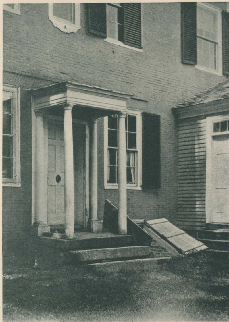
Detail of Side Porch.
