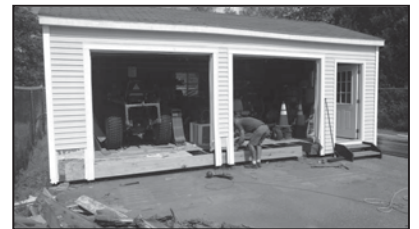
Bruce Sewell of Warren repairs a rotted sill on our tractor and mower building. The building was originally built by Steve Mills in 2003, and has held up very well except for some water intrusion that Bruce addressed around the roll-up doors. July 28, 2018.
