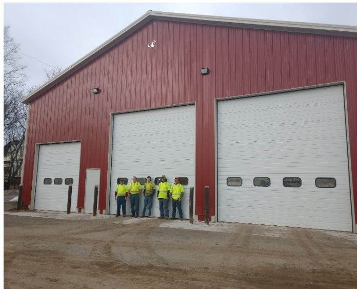
PICTURED ABOVE IS THE NEW HIGHWAY GARAGE
