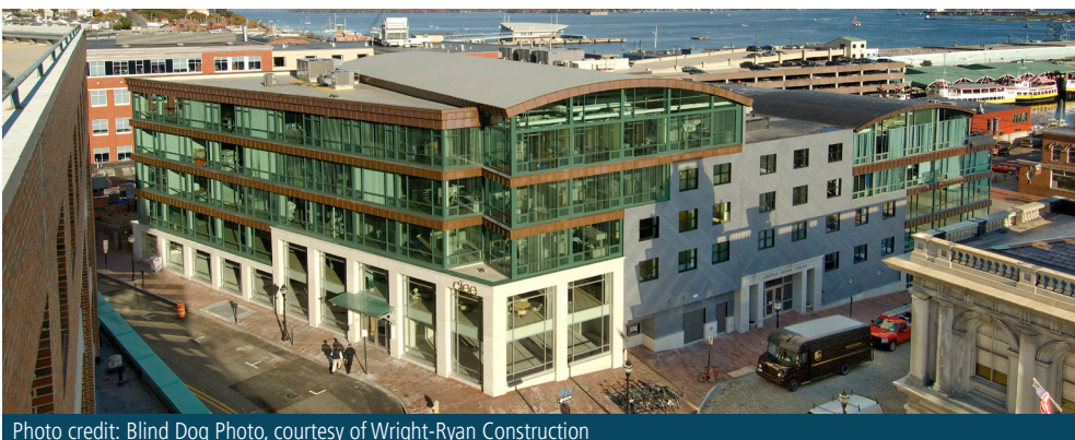
Photo credit: Blind Dog Photo, courtesy of Wright-Ryan Construction
