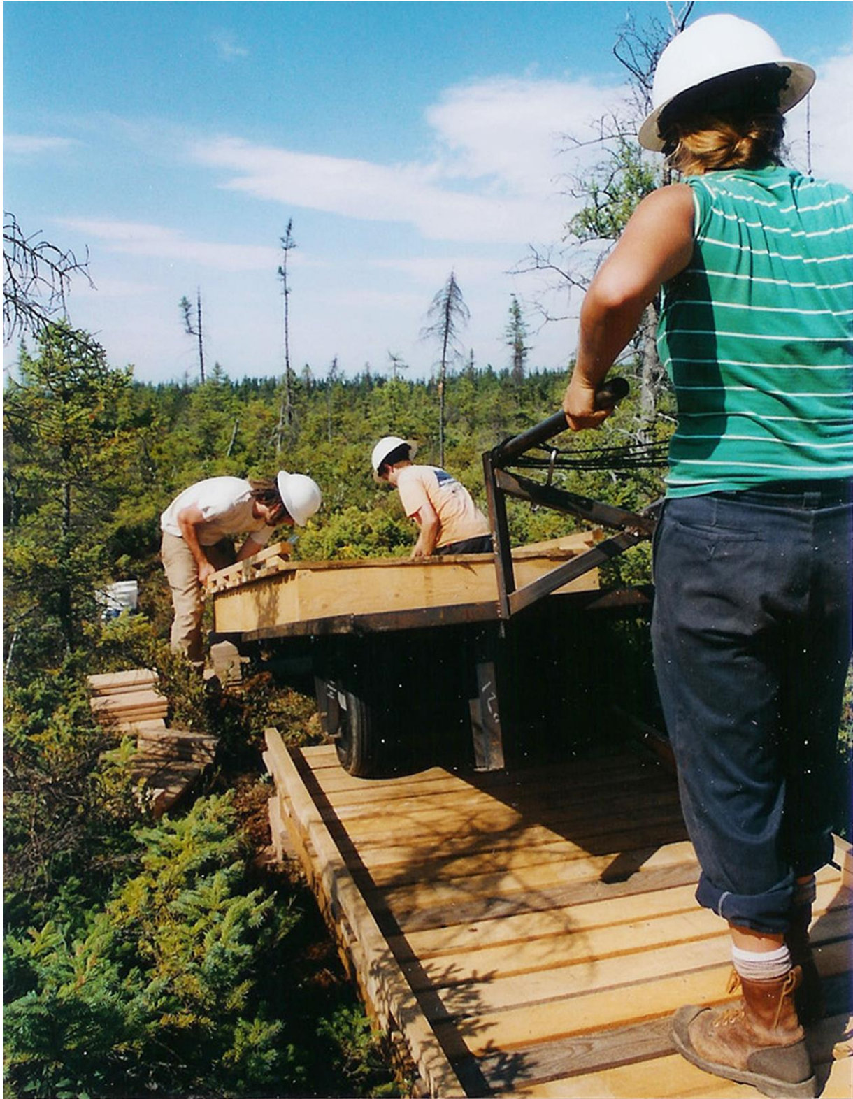
Fig. 20. MCC member tipping/sliding section off cart at end of incomplete boardwalk onto composite footings. Ron Lisnet UM photo.
