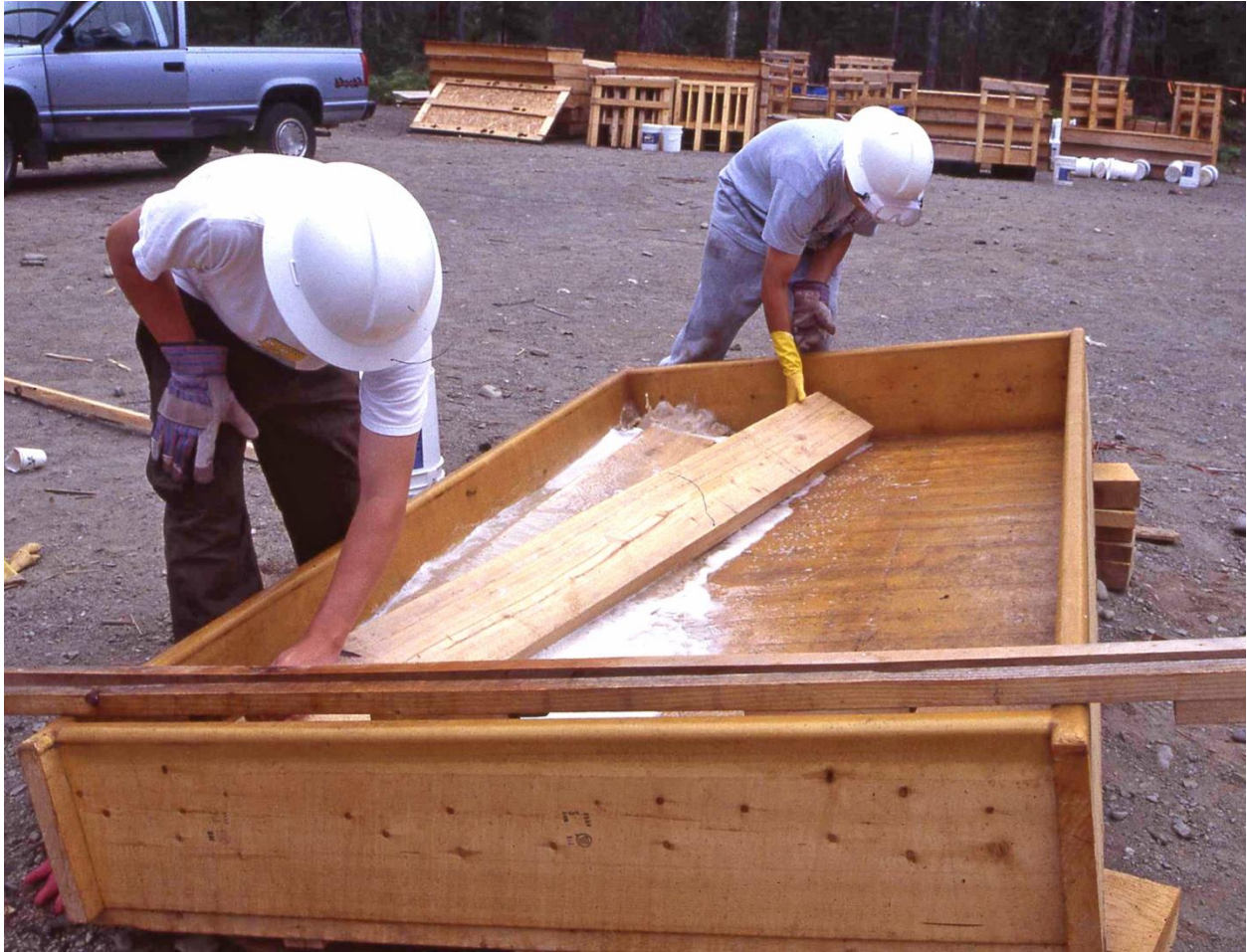
Fig. 16. Dipping section joists in wood-preservative in fiberglass-lined wooden “bathtub.” Components of interpretive stations (Fig. 8) appear in background along with full and empty 5-gallon buckets of wood preservative. Tom Hanson’s truck is in left background. Ronald B. Davis photo.
