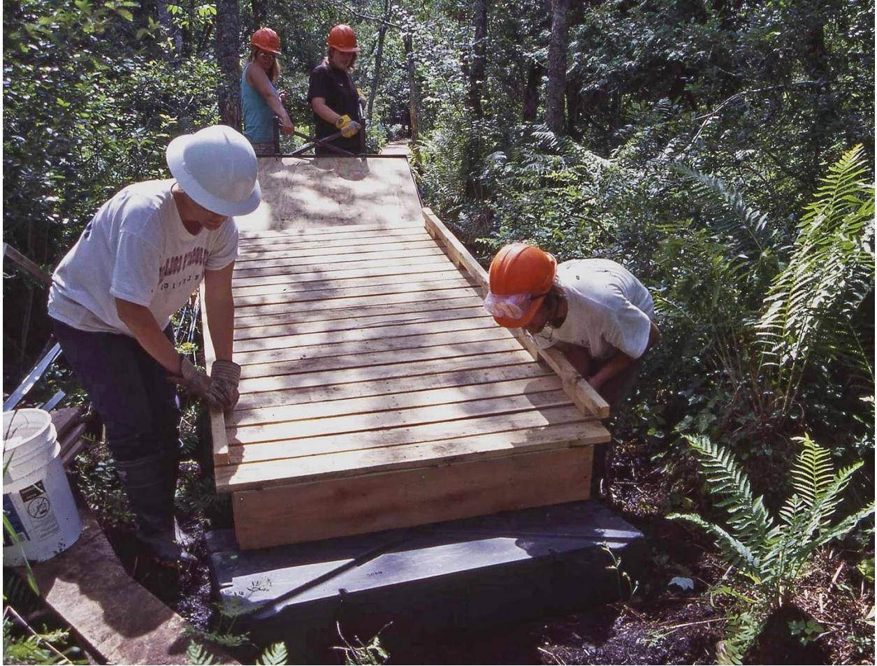
Fig. 21. Receiving section from cart at end of incomplete boardwalk and positioning it onto floats in mid-summer 2002. This location has standing water in spring. Ronald B. Davis photo.
