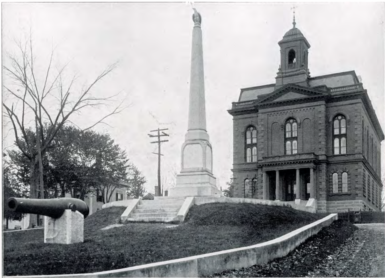
SAGADAHOC COUNTY COURT HOUSE, BATH.
