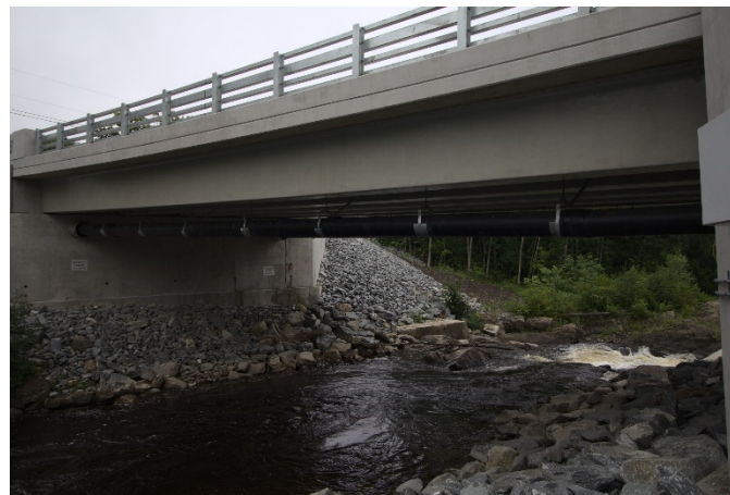
Figure 3. 22.9 m Span FRP Girder Bridge in Hampden, Maine, USA Constructed in 2020.
