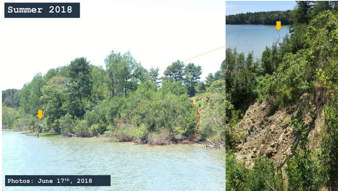
Figure 5.7 e. It was later observed that the portion of the bluff (thin red-dashed lines, center) between the LR 1 and LR 2 sub sites had failed. It retained much of its vegetation cover (still living, freshly foliated) and remained difficult to photograph; it would be difficult for a passerby to notice that an event had occurred at all. The displacement is more easily seen in the scarp upslope, behind the stand of young trees that were carried down. The yellow arrow marks a dead tree at the high-water line that can be seen in each image.
