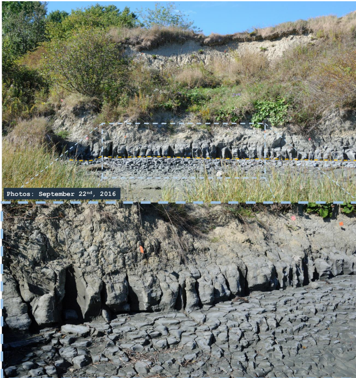
Figure 5.10 a. "Calving," or "Quarrying," of Dessicated Sediments from the Bluff Toe. Little River, Freeport, Maine, Sub-site LR 4. The bluff toe featured a blocky, quarried appearance that developed throughout the summer months. Note the significant under-cutting by concentrated erosion at the water line; the dry state of the Presumpscot Fm.; and the ubiquitous vertical jointing.
