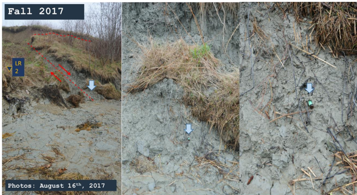
Figure 5.7 b. View from the LR 2 sub site. Showing toe creep of the failing block. Most of the painted rebar segments that were placed (on December 7 th , 2016) were eventually exhumed or lost in slides. The one seen here was engulfed by the advancing sediments.
