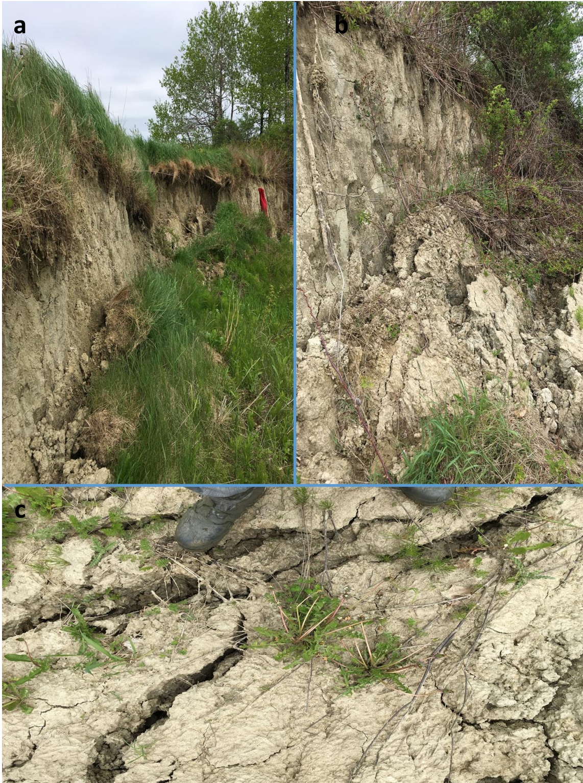
Figure 2.13 a-c. Mid-slope Slump Blocks and Tension Cracks. Breaks in slope behind slumped fault blocks (a, b), as well as associated tension cracks (c), present clear conduits for surface water to get into slip-planes and increase sensitivity to further slope failure.
