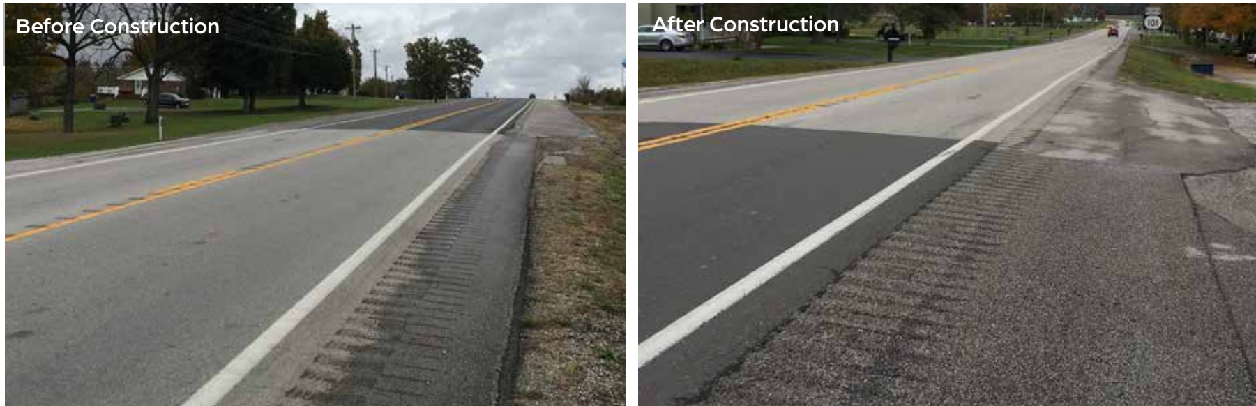
Figure 3.14 KY 101 After Construction
