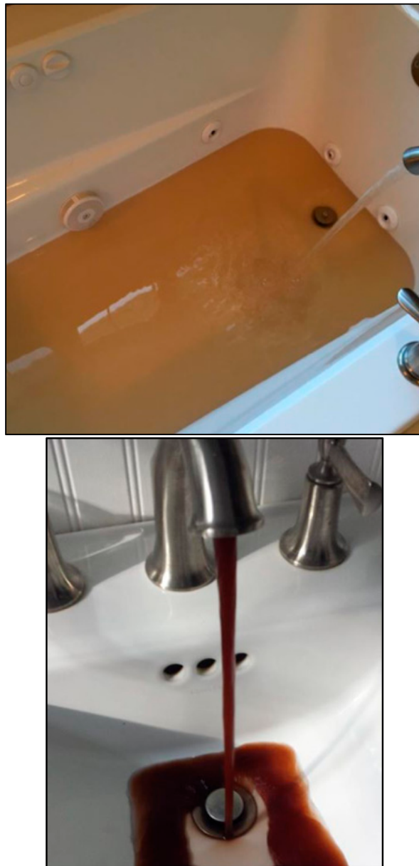
Figure 2. Photos of discolored tap water in Holliston homes, posted on Facebook ® by Holliston residents.
