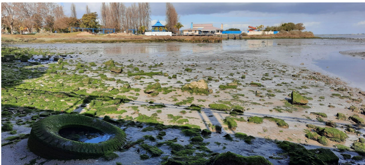
High organic material conditions at the sewer outlet, Bareiro
