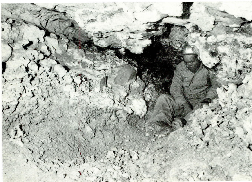
Fig. 2. Partly mucked-out solution channel at end of mucked-out cavern.
