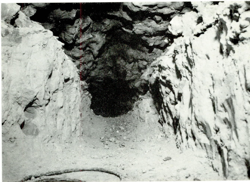
Fig. 1. End of mucked-out cavern beyond which two solution channels extend approximately 50 feet.
