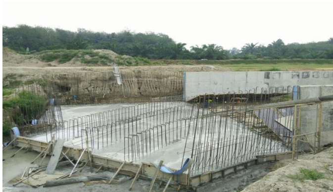
Retaining Wall Kanan
