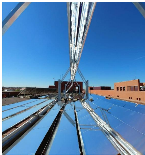
Fig. 1.3. Linear concentrating solar collectors. Parabolic trough collector PTC working principle (a), example (c). Linear Fresnel collector working principle, with an evacuated receiver and secondary reflector (b) and example (d).
