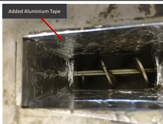
Figure 4-23 The added aluminium for smoothness of surface
