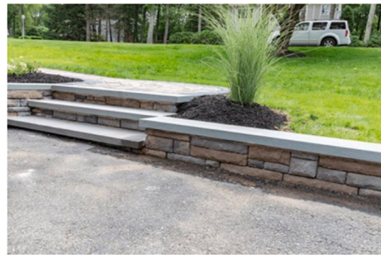
(b) Solidia concrete blocks
