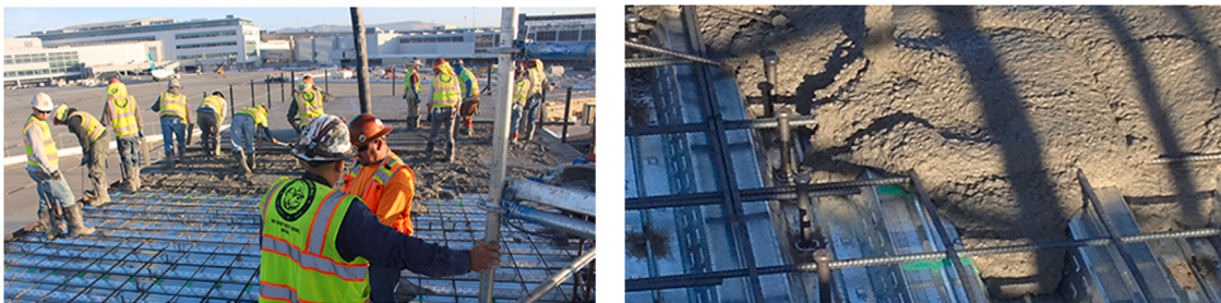
Fig. 19. Placement of Blue Planet's concrete at the San Francisco International Airport [168].
